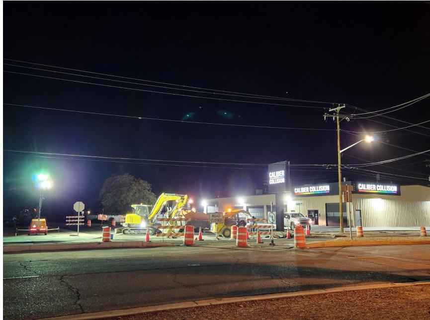
Storm sewer improvements at 29 ¼ Rd.
