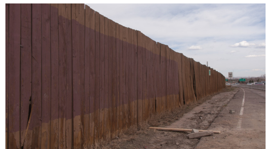
Old fence pickets donated to create new outfield fence
