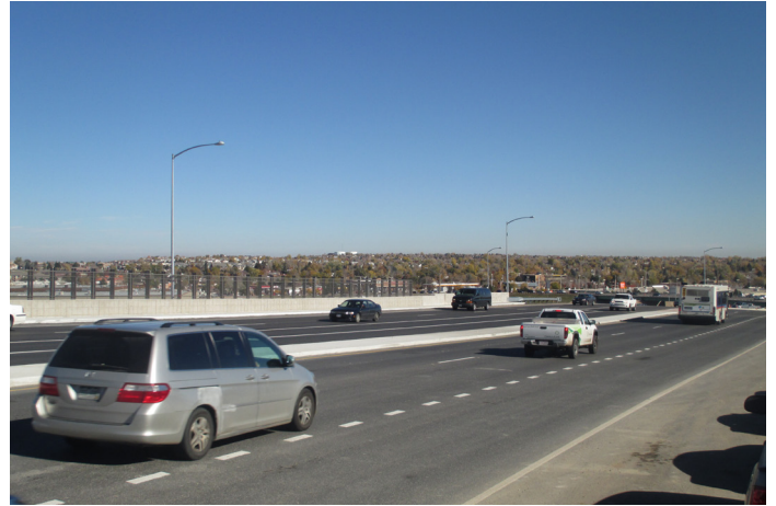
Cars on the new Wadsworth Parkway bridge
